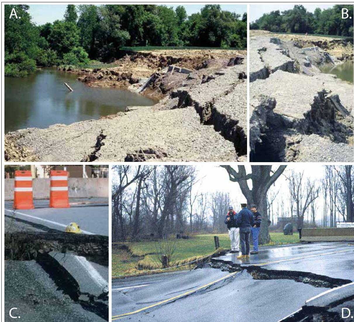
Figure 5. Surface effects related to Retsof Mine roof collapse. A and B) Partially water-filled solution collapse dolines above the region of yield pillars in the Retsof Salt Mine. C & D) Subsidence-related roadbed collapse on Route 20A (images downloaded from < <http://www.rcsiweb.org/gallery.html>> on Dec 6, 2016).
